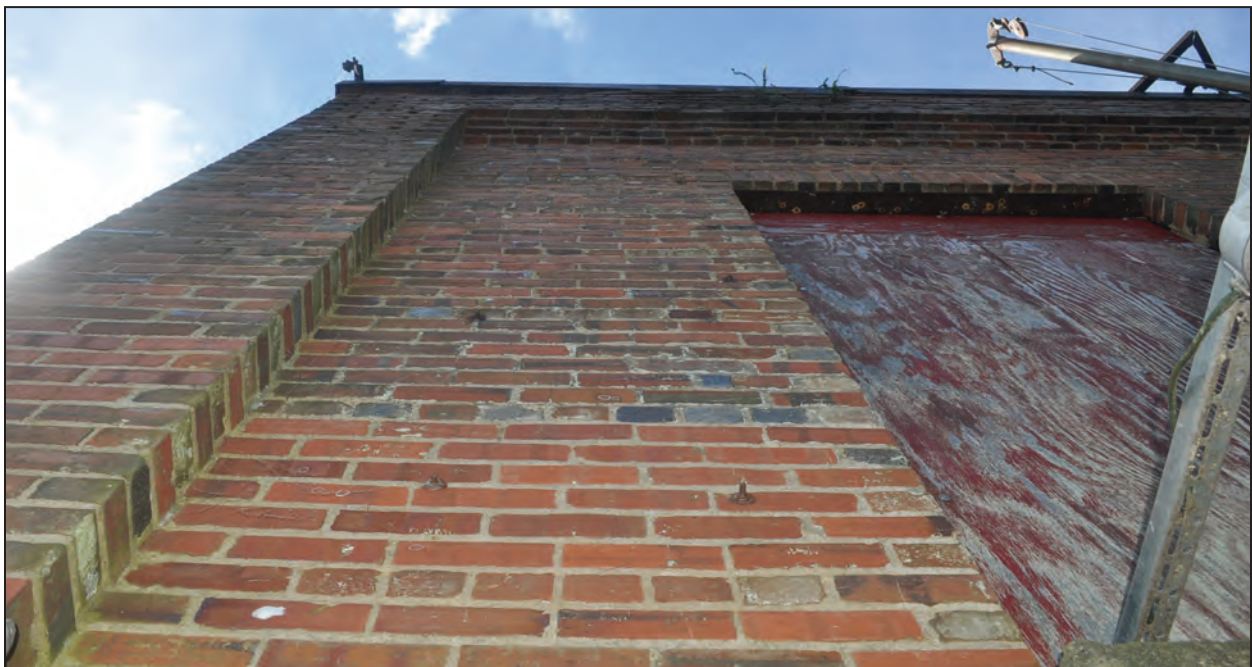
B. North Wall of Powerhouse
