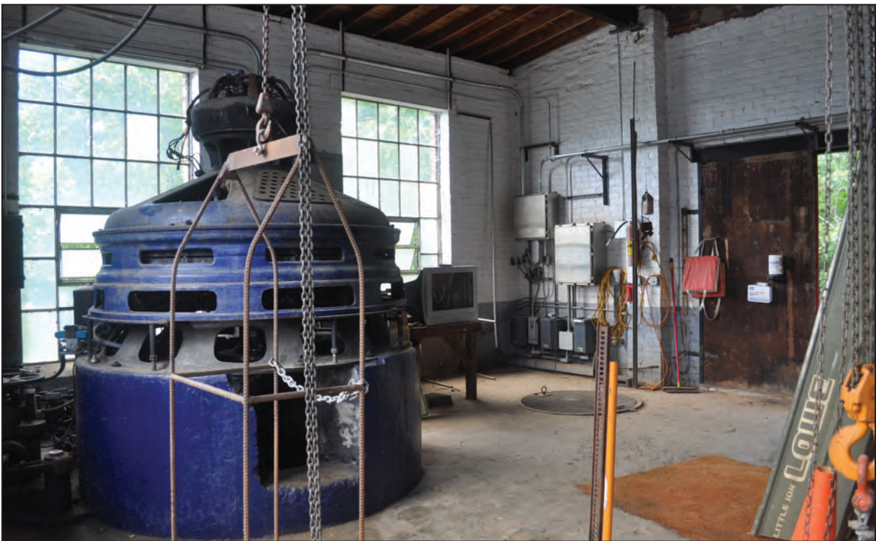
B. Interior of Powerhouse Looking Southwest
