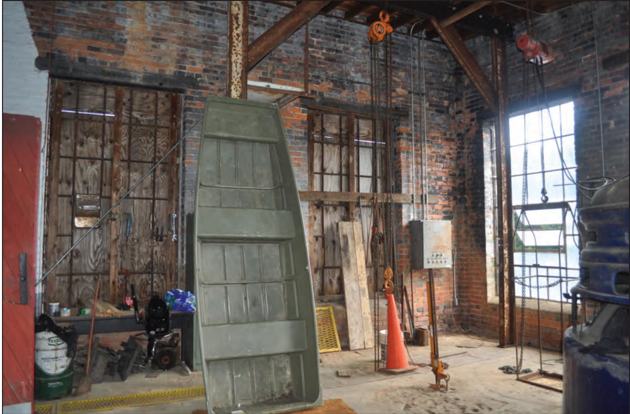
B. Interior of Powerhouse Looking North
