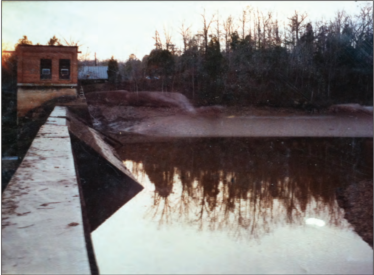
Figure 10. Historic Photograph Showing Upstream Sides of the Circa 1925 and the 1944 Dam Sections
