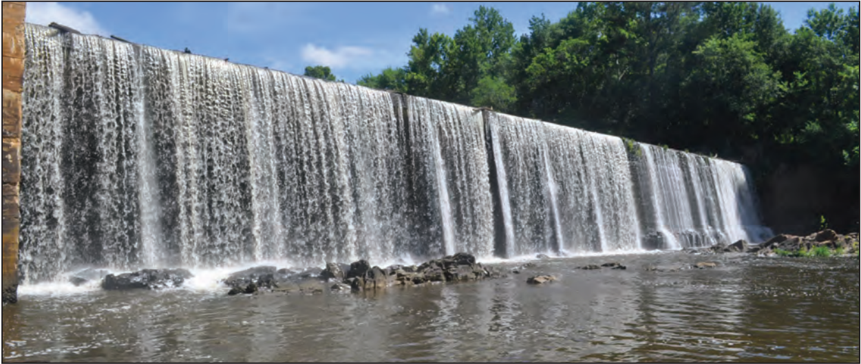
A. Downstream Side of Dam Looking Northeast from South of Powerhouse
