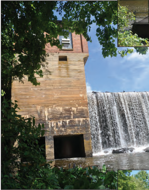
B. Powerhouse Looking North
